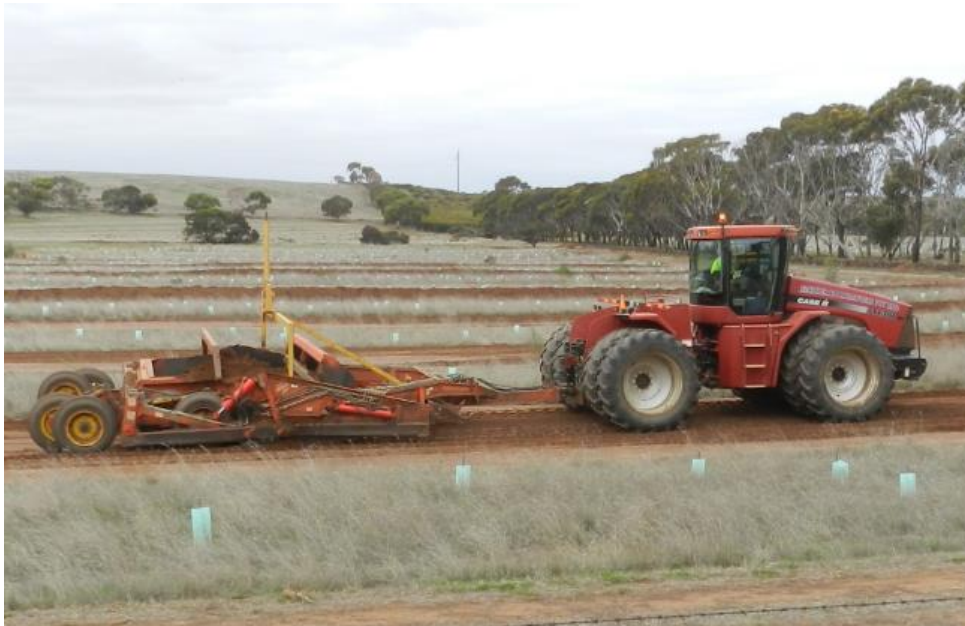
Figure 23: Picking up windrowed topsoil with a Case IH/ Land Plane combination – 141 Mine Rd.
